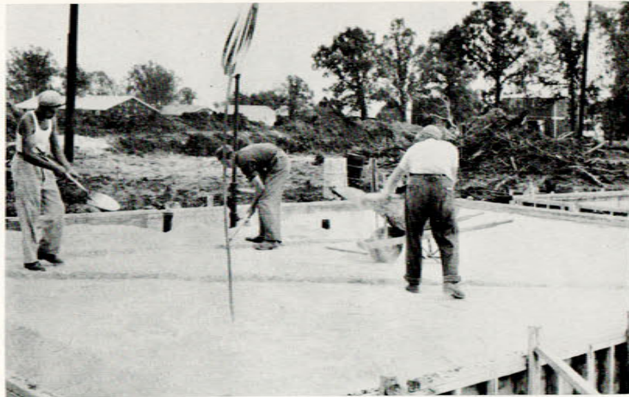
Preparing of Slab Foundation for the pouring of concrete
