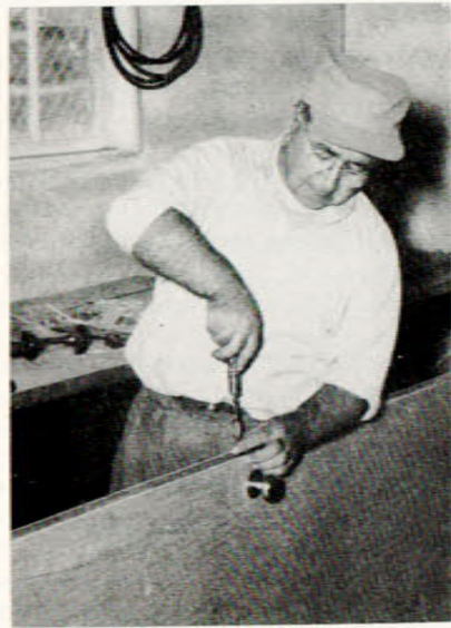
Carpenter putting hardware on one of the mahogany doors.
