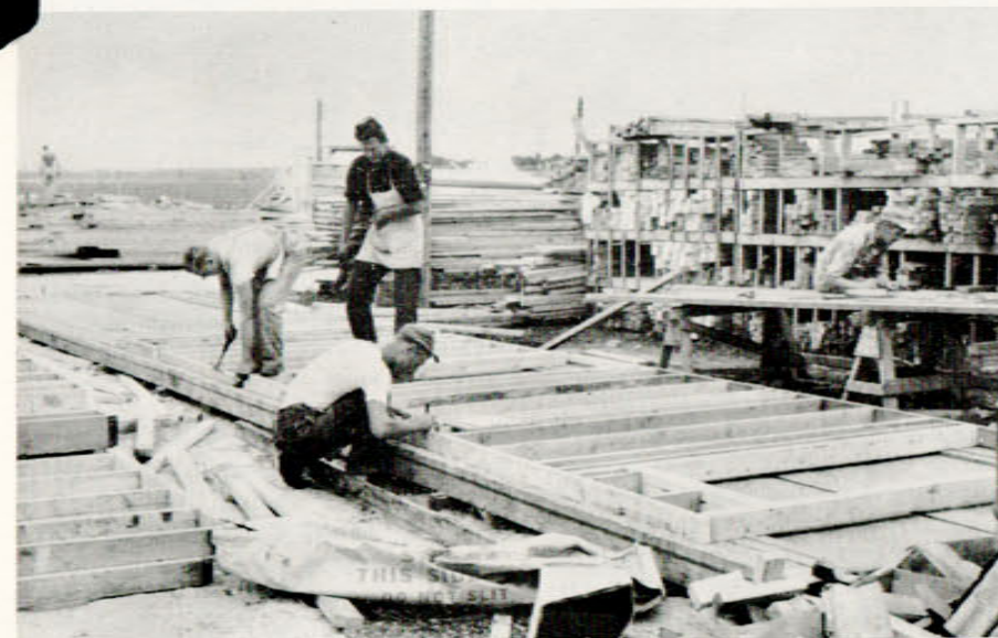
Side wall being pre-fabricated on jig and template
