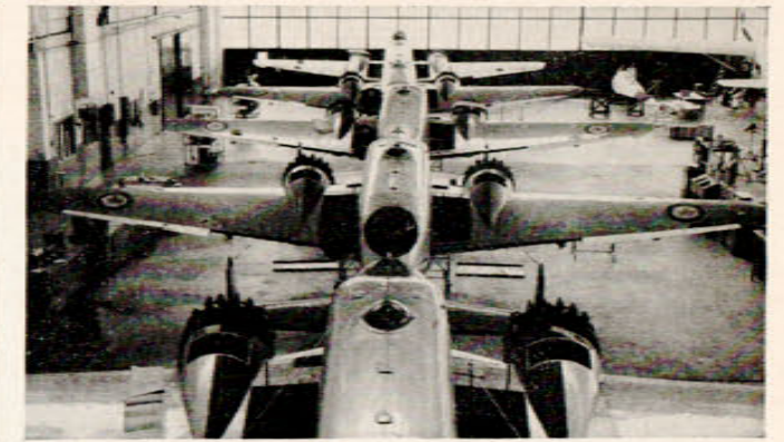
Bristol helps keep the RCAF flying through its part in the RCAF's CAIR (Calendar Aircraft Inspection and Repair) program. Contracts are held for regular checks on RCAF Beech Expeditors and CF-100 interceptors in Western Canada.
