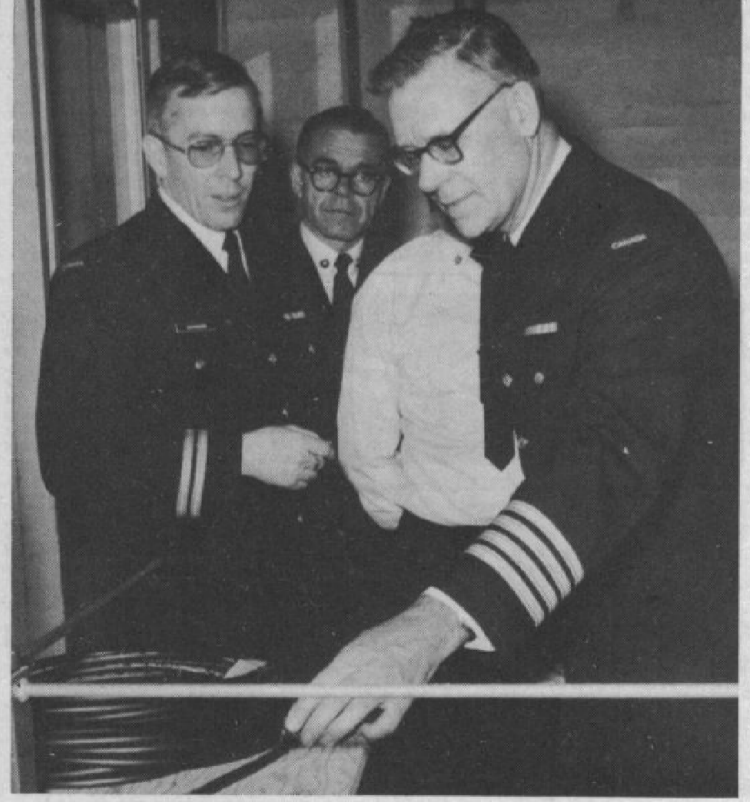
CAPT JOHNSON, MWO H. Dyrda and the Commander discuss the installation of a locally produced antenna during Col Wylie's visit to the former Ground Telecom Section, now a part of 733 Communication Squadron.
