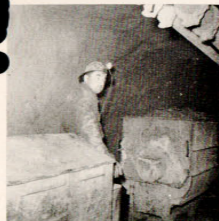
The "work horses" of the mine. Small ore train used for removing blasted muck from the tunnels and eventually to the surface.
