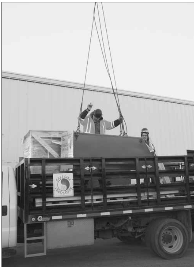
The dust collector is craned off a delivery truck in pieces for assembly onsite on November 10. Photo: Bill McLeod, Voxair Manager
