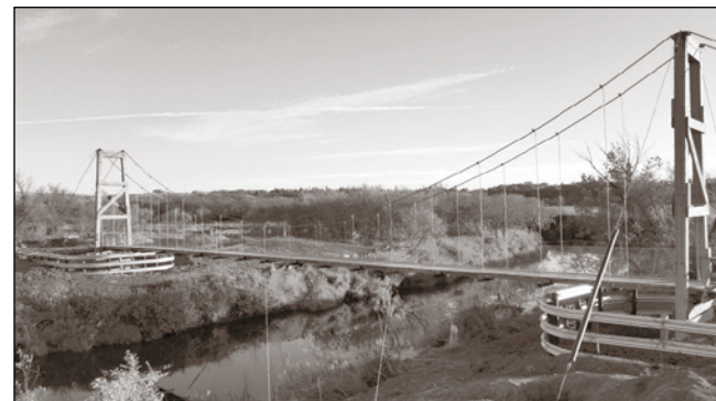
The bridge is a timber construction suspension bridge with a span of 44m and is funded by the Trans Canada Trail, the City of Moose Jaw and the Wakamow Valley Development Fund and will serve to connect Moose Jaw and complete the Trans Canada Trail 100% in the province of Saskatchewan.
