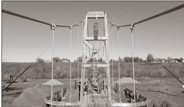
The bridge towers are a heavy timber construction and are 10m in height. The bridge span is 44m and the walkway is 2m wide.
