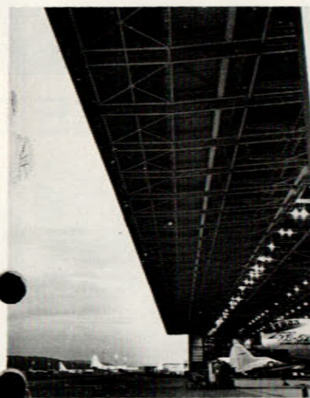
Thirteen vertical lift doors on Boeing Airplane Company's new multi-million-dollar flight test hangar at Seattle are shown fully up, revealing the largest unobstructed doorway in the United States. The doorway measures one-sixth of a mile in length and is 65 feet high. The hangar itself is 785 feet long, 200 feet wide and 90 feet high. It can comfortably house five Boeing B-52 Stratofortress heavy bombers and will be able to accommodate airplanes of the future with wingspans up to 300 feet. —Boeing Airplane Company Photo.
