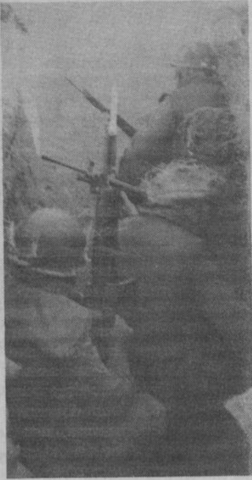
The dirty job of "trench clearing". Photo by Cpl Gomm
